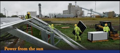
**Above** | Contractors build the first portion of Corn Belt Power's new solar array at Wisdom Station Oct. 10. The 150-kilowatt system should be complete in the beginning of 2020.
